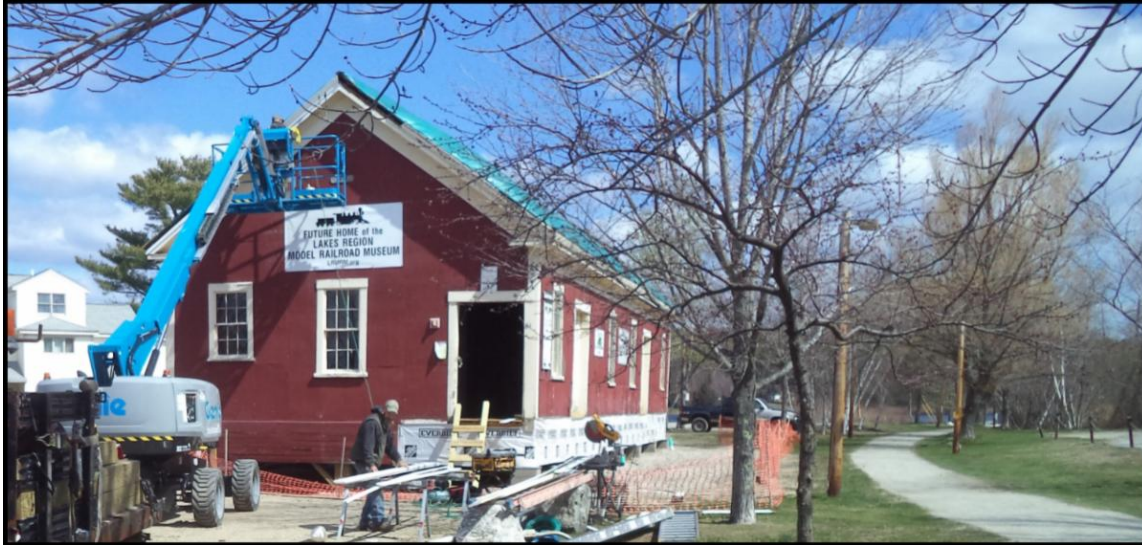
Rehabilitation work is well underway at the Wolfeboro Freight Shed
