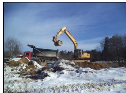
Dam construction is underway to
